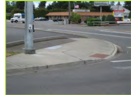
New Curb Ramps with Truncated Domes
