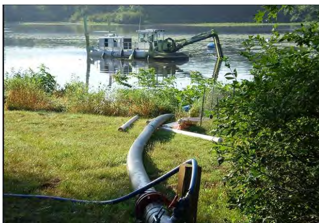
Figure 5-1. Hydraulic dredging (MSA Professional Services)
