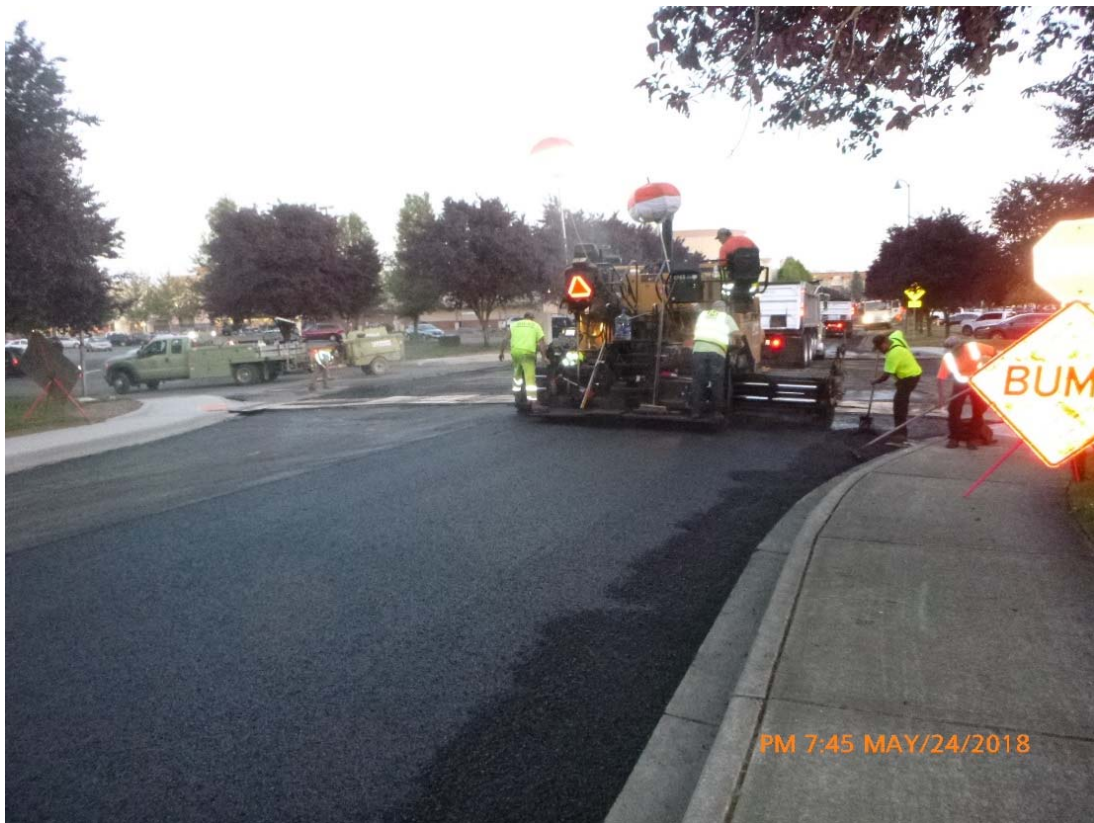
Roadway grinding and Hot Mix asphalt overlay of the existing roadway.
