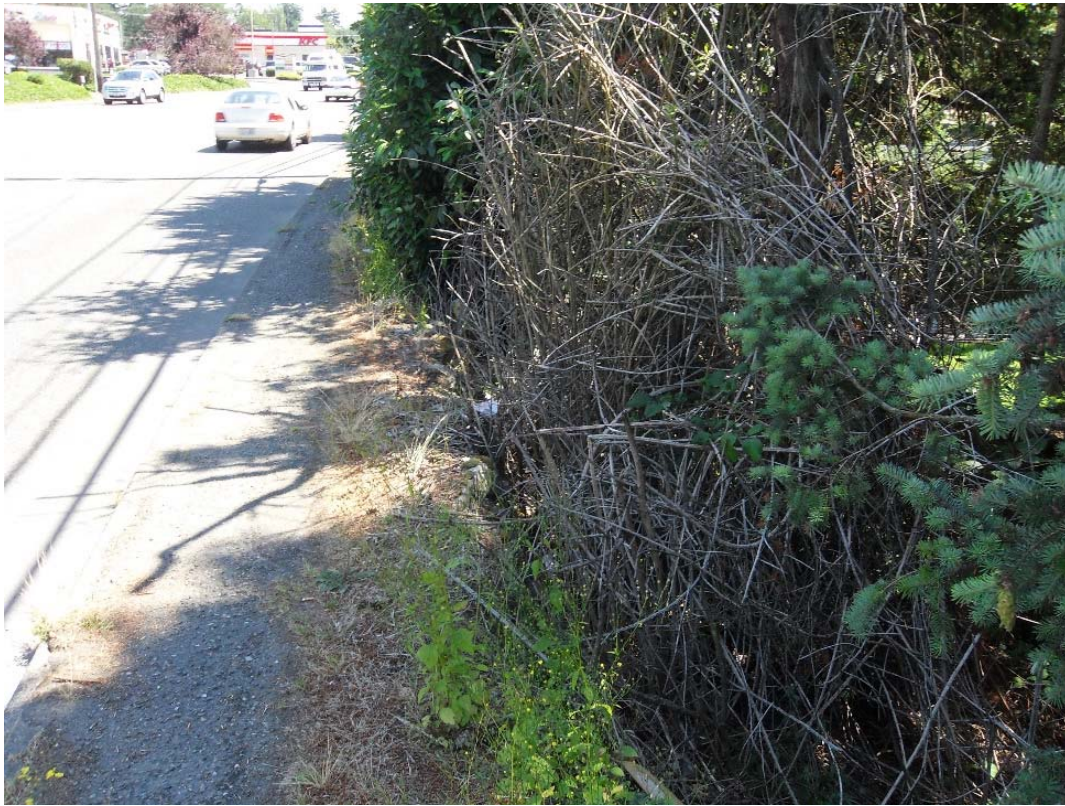
Existing Condition: showing need for overlay, curb and gutter, and sidewalk. (Steilacoom Blvd. looking east on the south side of the road between Phillips Rd. and Weller Rd.)
