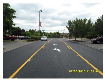
The project included upgrading as necessary, all abutting sidewalks to meet ADA requirements, performing all road surface preparation work from pavement patching, to curb lane and lane grinding to street sweeping to tack coating the existing pavement. This is followed by laying a 2-inch thick asphalt overlay over the entire roadway surface from Gravelly Lake Drive to 108<sup>th</sup> St. and after appropriate curing time, installing new lane markings.
