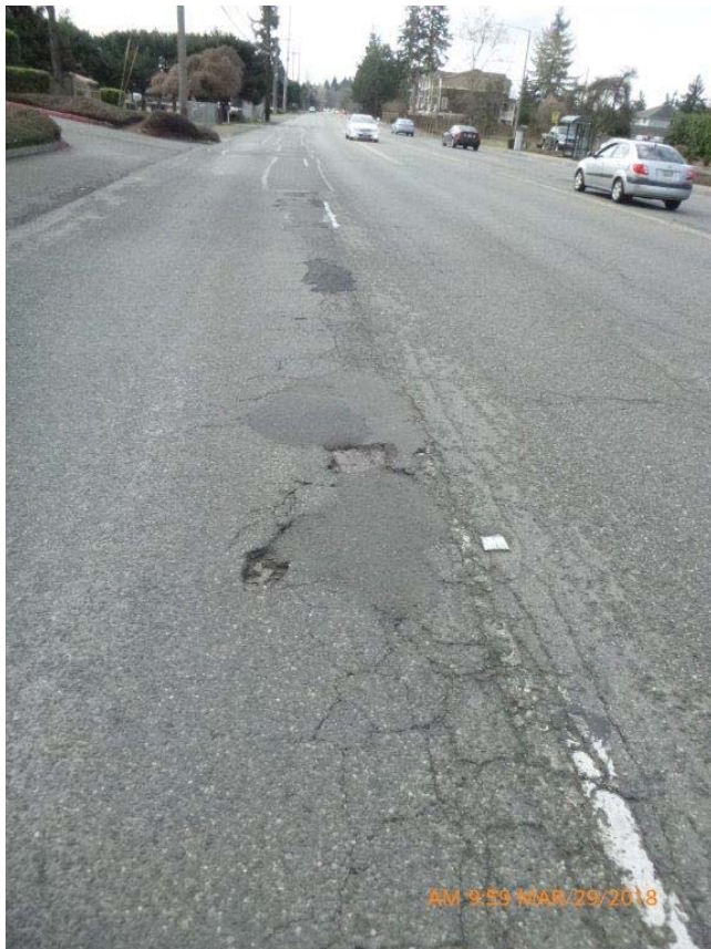
Current condition of Lakewood Drive, full depth pavement failure and roadway patching.
