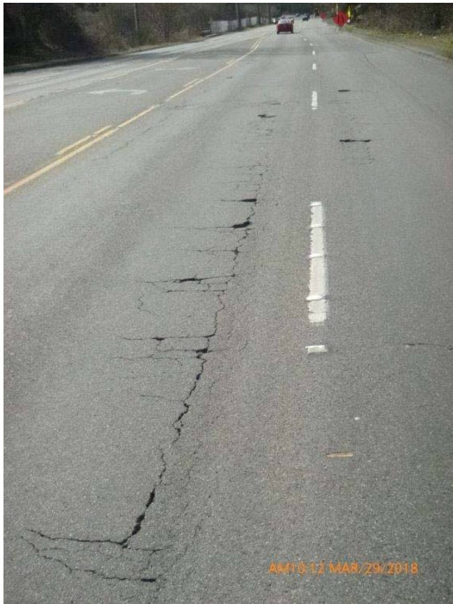
Current condition of Lakewood Drive, full depth pavement failure in wheel paths.
