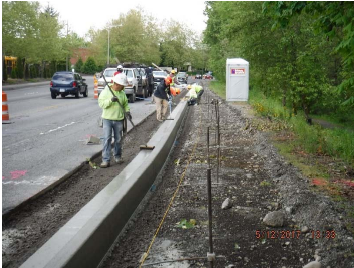
New curb and gutter, Seeley Lake side of Lakewood Dr.
