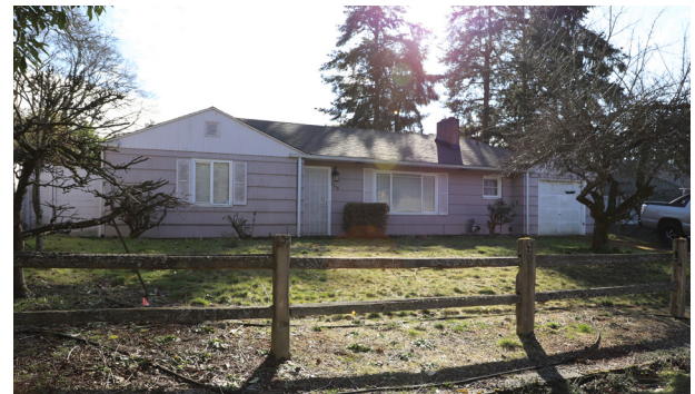
5618 Mt. Tacoma Drive, a ranch house.
