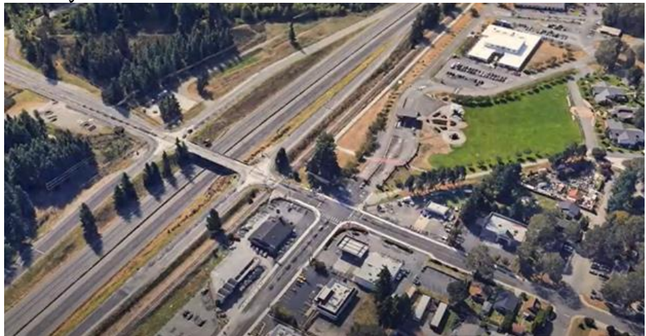
Figure 1 – Berkeley/I-5 Intersection Prior to Reconstruction
