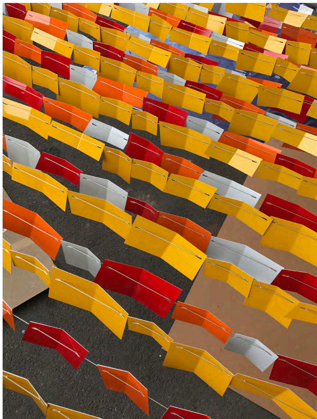
On the street side, prismatic film on aluminum reflectors create excellent internal glow through car headlights.
