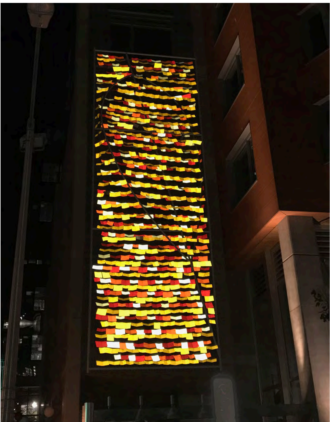
On the street side, prismatic film on aluminum reflectors create excellent internal glow through car headlights.
