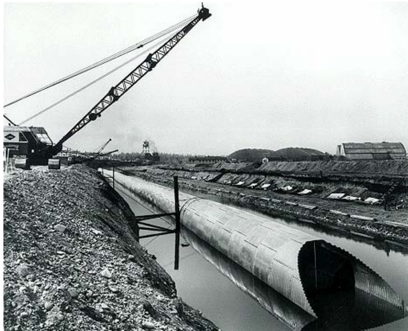
Figure 14. The McChord Airbase channel dredged in 1938 with one of the two 12-ft diameter culvert pipes, 1400 ft long, rolled into place, courtesy of the Tacoma public Library
