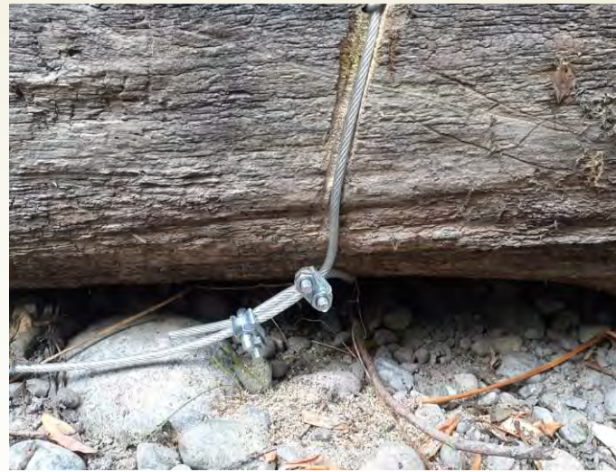
Used a cable and 16" screw anchor.
