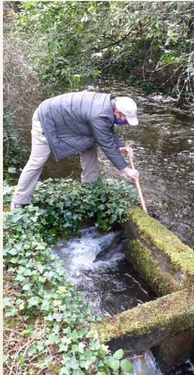
Darin Masters, WDFW, works to unplug ladder opening.
