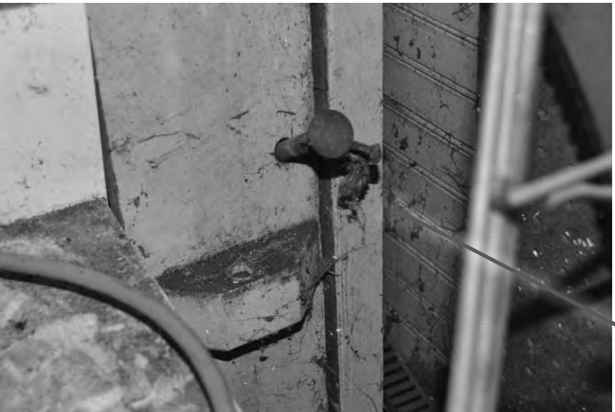
7 HISTORIC LOCKING BOLT AND WOOD HOLDER. VERIFY ALLOWS DOOR IN NEW CONFIGURATION TO BE OPERATIONAL
