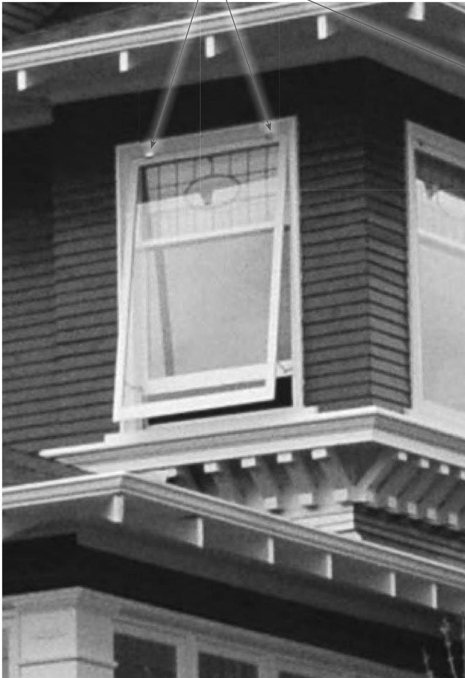
SOLID STEEL HEAVY DUTY STORM WINDOW HANGER, SATIN BLACK FINISH, TYP 2 PER WINDOW
