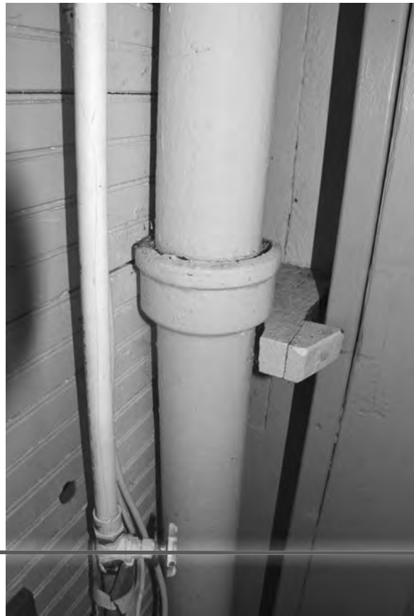
1 THE HISTORIC SANITARY TAND WATER SUPPLY TO THE DEMOLISHED UPPER FLOOR SANITARY DETERMINED TO BE NON-FUNCTIONAL: RESTORE AS HISTORIC ARTIFACT. IF WATER SUPPLY SERVICABLE, PATCH & REPAIR FOR NEW USE, IF NOT: RESTORE AS HISTORIC ARTIFACT.
