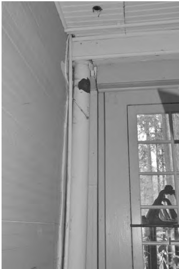
1 THE HISTORIC SANITARY TAND WATER SUPPLY TO THE DEMOLISHED UPPER FLOOR SANITARY DETERMINED TO BE NON-FUNCTIONAL: RESTORE AS HISTORIC ARTIFACT. IF WATER SUPPLY SERVICABLE, PATCH & REPAIR FOR NEW USE, IF NOT: RESTORE AS HISTORIC ARTIFACT.
