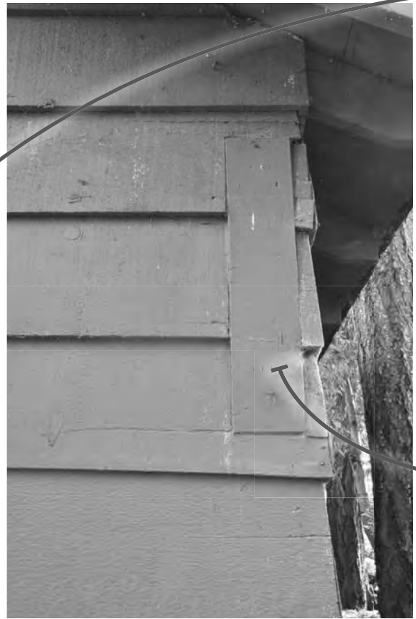
10 RETAIN EXTANT PORTION OF HISTORIC KNEE BRACKETS IN SITU. RECONSTRUCT EXTANT BRACKETS & FABRICATE NEW BRACKETS BASED ON EXTANT, VISIBLE IN MULTIPLE LOCATION, TYP
