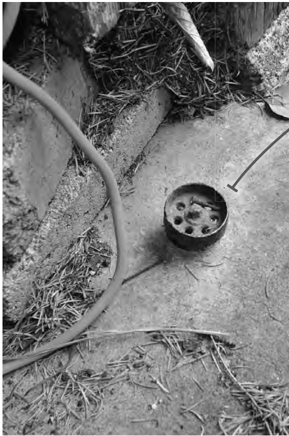
9 RESTORE SLIDING DOOR FLOOR GUIDES, AS PRACTICAL, TYP
