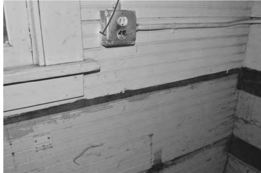
16 REPAIR SURFACE OUTLETS - REMAIN EXPOSED, TYP
