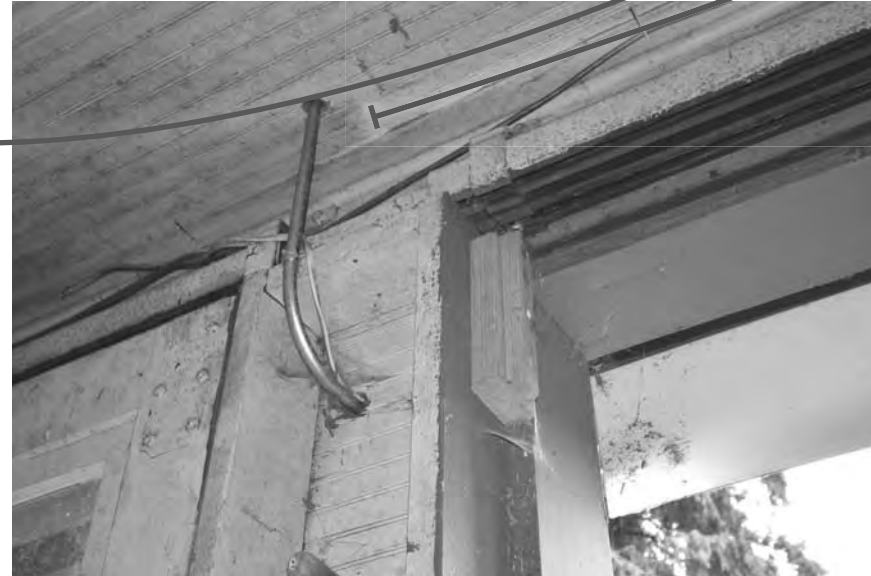
14 EXPOSED CONDUIT VERIFY FUNCTIONALITY - REMAIN EXPOSED, TYP
