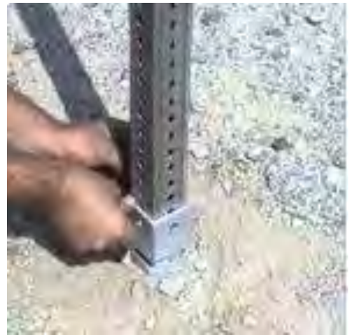
Poles will be cemented into the ground
