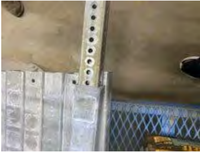
Example of the telespar inside the heavy-duty anchor
