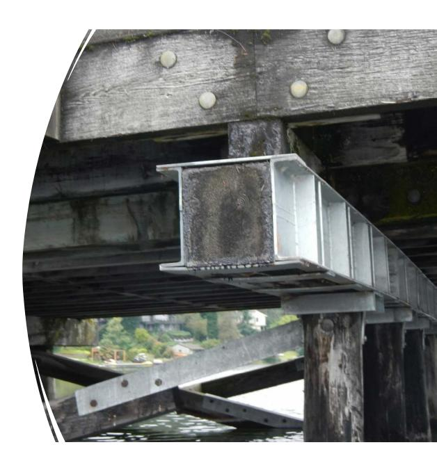
This option includes work performed to replace the pile caps which currently have a critical finding rating. Without replacing these caps, the bridge cannot reopen. Caps on Bents 6, 12, 15, 16, 21, 33, 40, and 43 are at the point where the beams can no longer support adequate weight to keep the bridge open.
