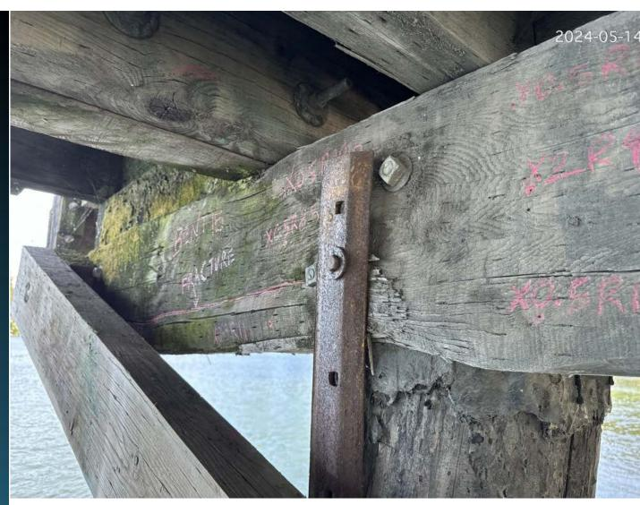
Cap is pulling the deck down in this condition, causing harm to surrounding members
