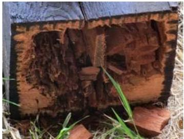
1/2" Shell thickness in Pile Cap 15 caused a 1.5" compressive failure. Photo to the left shows the compression on the cap of Bent 15 on May 14, 2024. Photo above is a representation on the interior condition of the pile cap.
