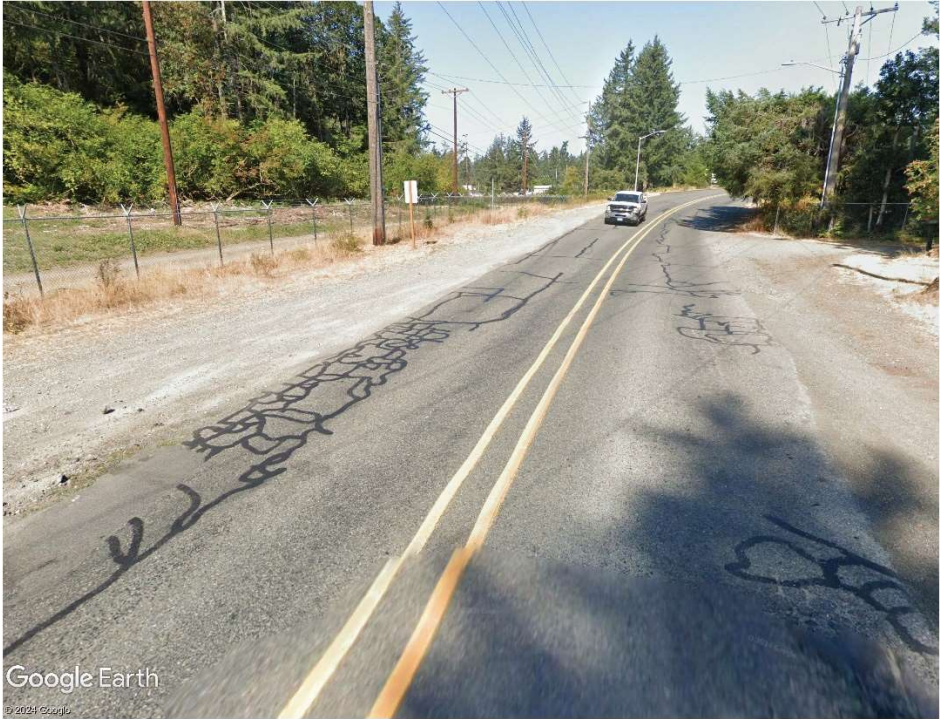
Before – Image Date April 2018 (Credit: Google)
