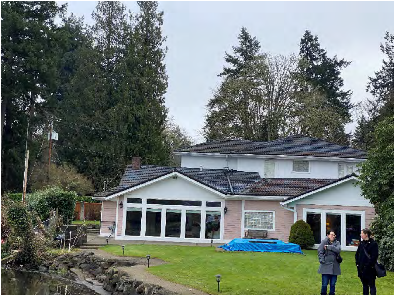
VIEW OF REAR ELEVATION
