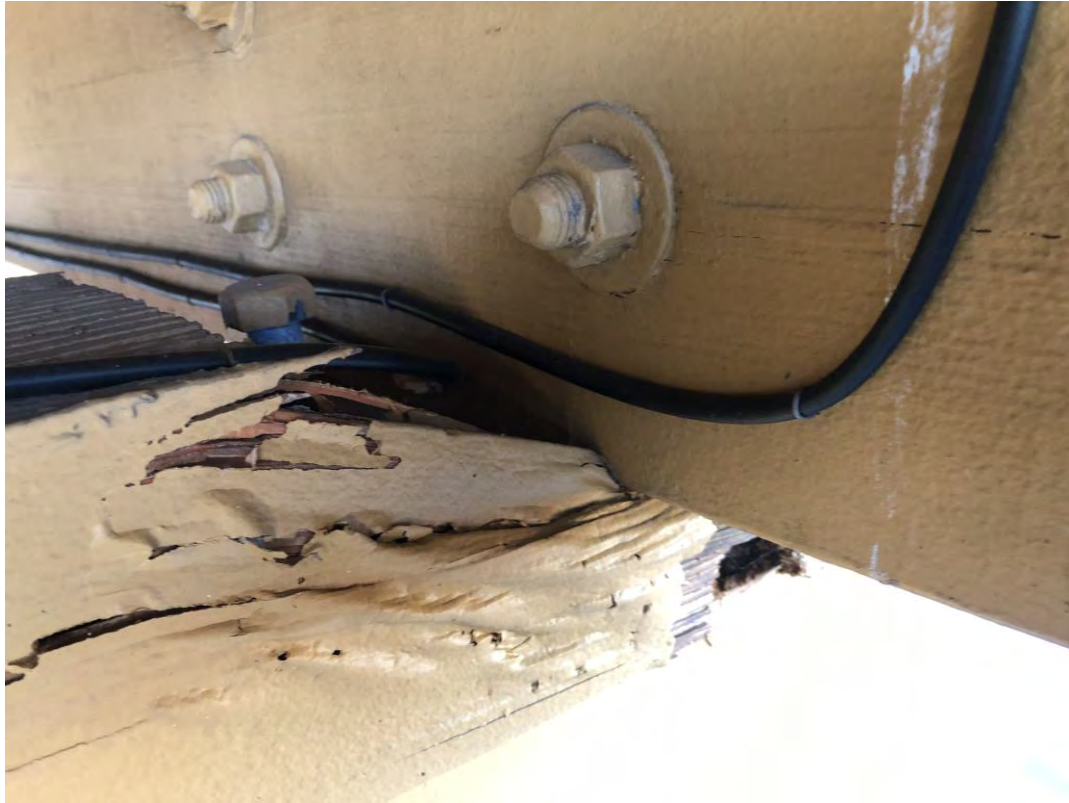
Low roof – Northeast end of building
