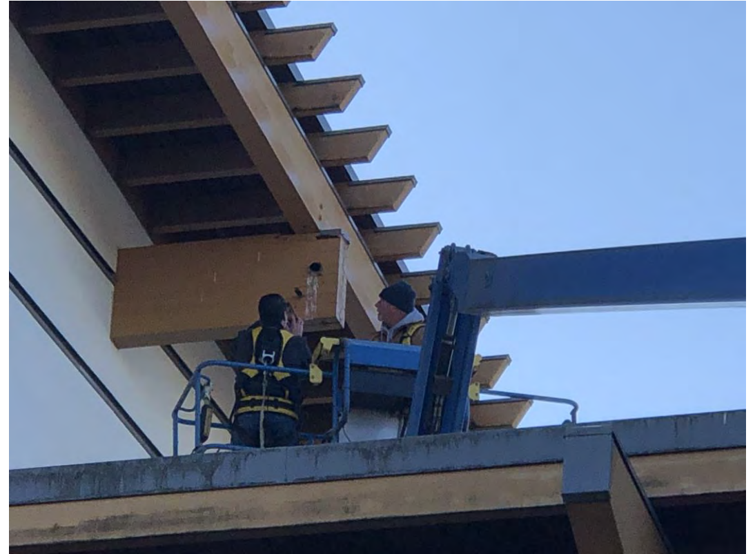
High roof – Northwest end of building
