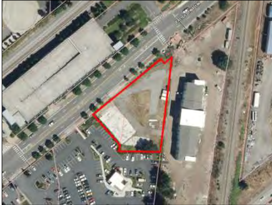
SE SIDE OF PACIFIC HIGHWAY SW, EAST OF BRIDGEPORT WAY
