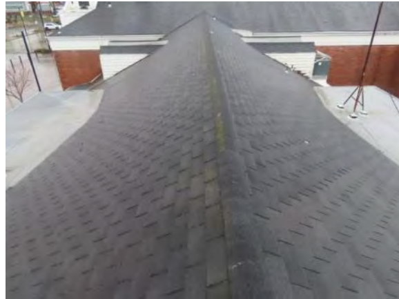
Pitched Roof of Building
