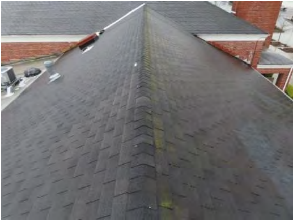
Pitched Roof of Building
