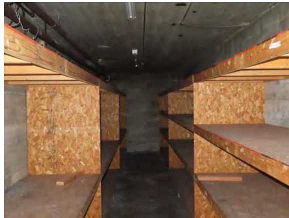
Basement Storage Area
