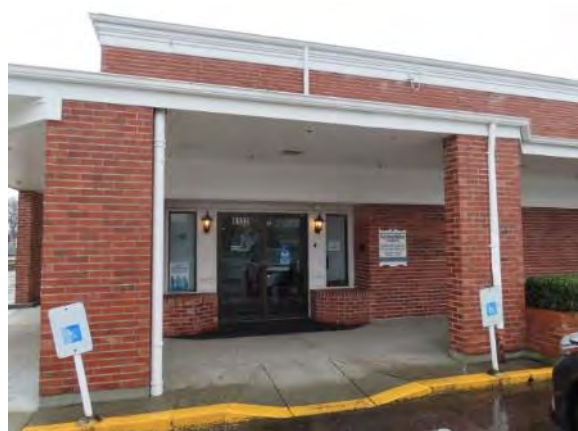
West Side of the Buildings
