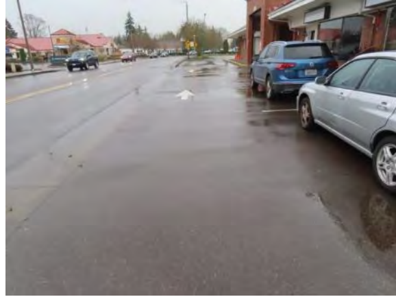
South Asphalt Parking Area
