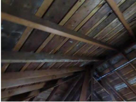
Typical Roof Framing
