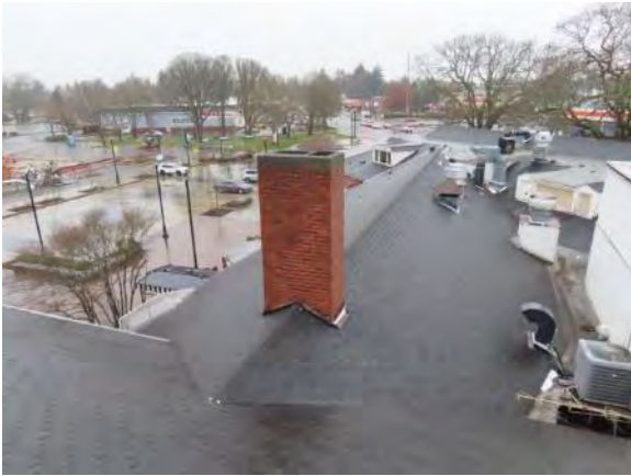
Pitched Roof of Building
