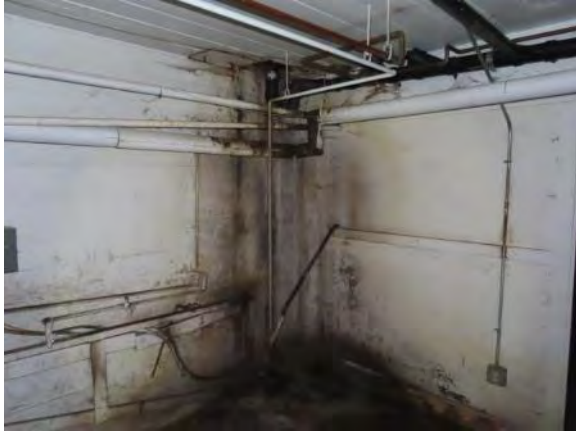
Concrete Foundation Walls
