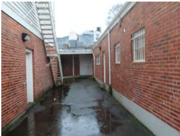
Interior Courtyard Facing Walls
