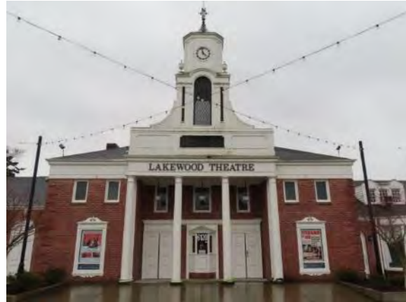
North Side of the Theater
