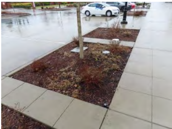
North Planter Bed and Concrete Sidewalk
