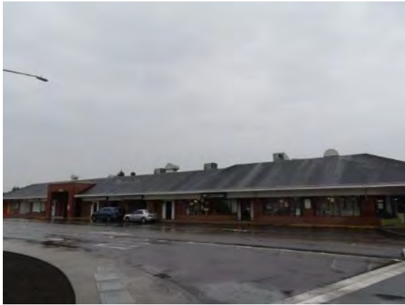
South Side of the Buildings
