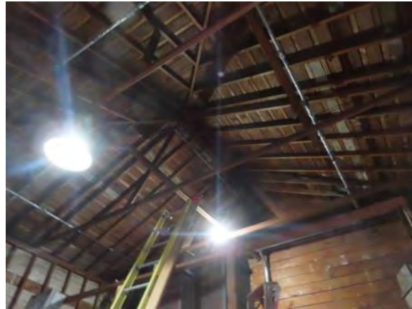
Typical Roof Framing
