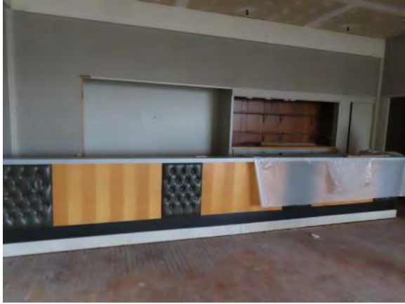
Abandoned Restaurant Bar
