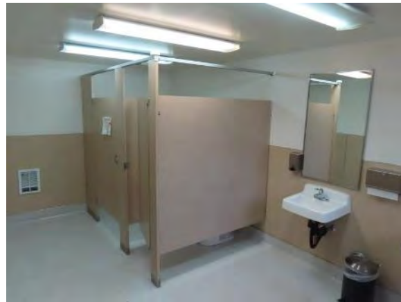
Unit 6209 Typical Restroom
