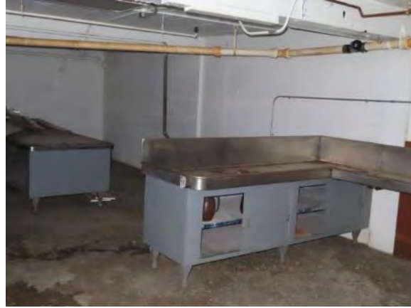
Concrete Foundation Walls
