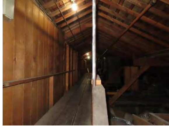
Typical Roof Framing
