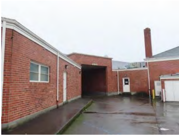
Interior Courtyard Facing Walls
