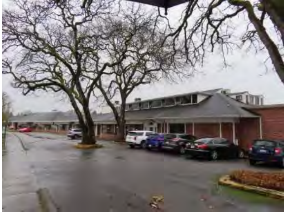
East Side of the Buildings
