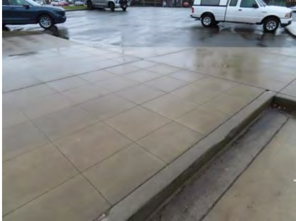
North Concrete Sidewalk
