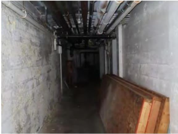
Concrete Foundation Walls
