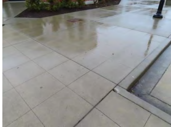
East Concrete Sidewalk
