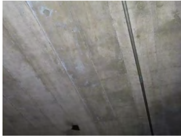
Concrete Foundation Walls
