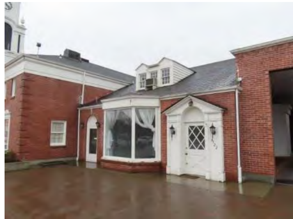
Apartment Entrance at the North Side
