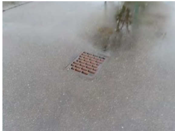
Typical Storm Drain in North Parking Lot
