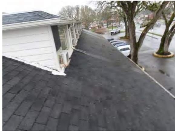
Pitched Roof of Building
