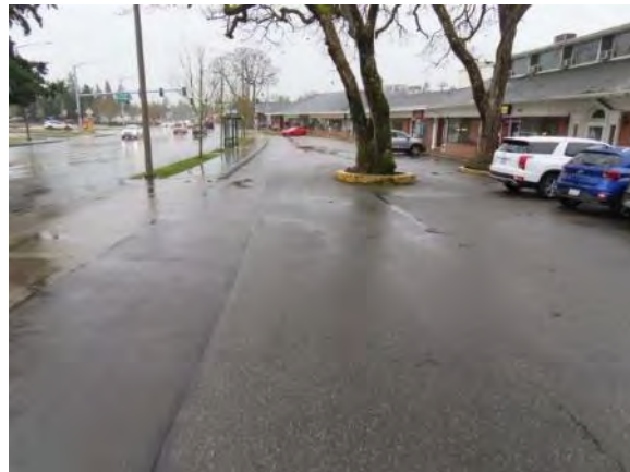
East Asphalt Parking Lot
