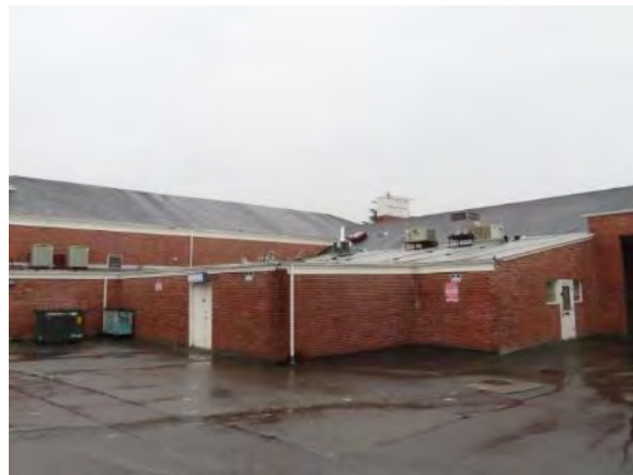
Interior Courtyard Facing Walls
