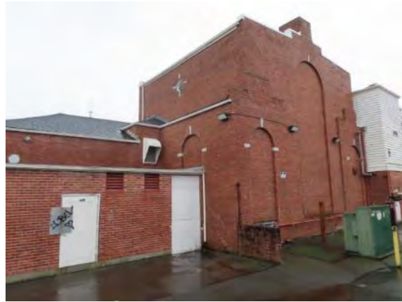
Interior Courtyard Facing Walls
