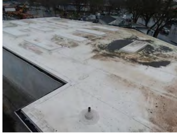
Flat Roof of the Theater Surfaced with PVC Roof Surfacing
