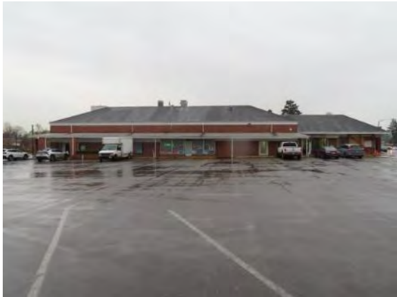
West Side of the Buildings
