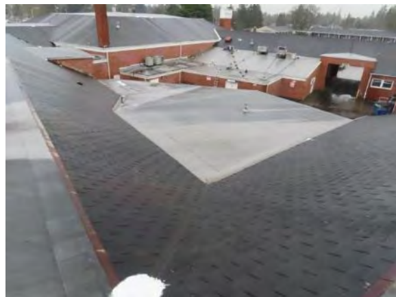
Modified Bitumen Torch-Applied Roof Surfacing on Low-Slope Areas of the Roof
