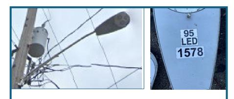
Pictured above is a City of Lakewood Owned streetlight installed on a wooden telephone pole (left). These lights often have a tri-bulb set up and have numbers somewhere on the luminaire head (right)
