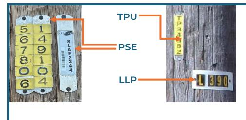
These are some examples of the pole ID tags you will see across Lakewood. PSE tags (left) come in two forms, one is two horizontal sets of six-digit numbers and the other is vertical tag with starting with "SLA". TPU tags (upper right) typically have 5 digits and begin with "TP". LLP tags are 3 digits and have an "L" at the beginning.
