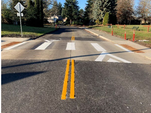
Onyx Drive ADA Improvements at 97 th Ave. SW
