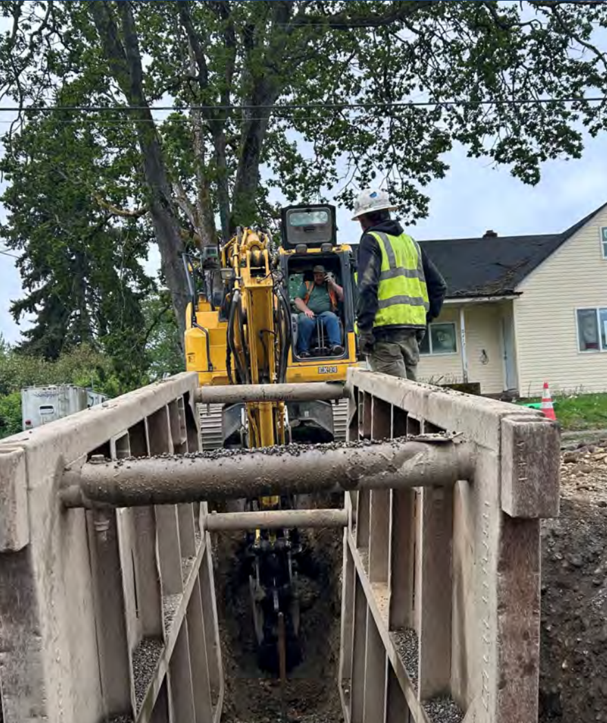
Sewer extension construction
