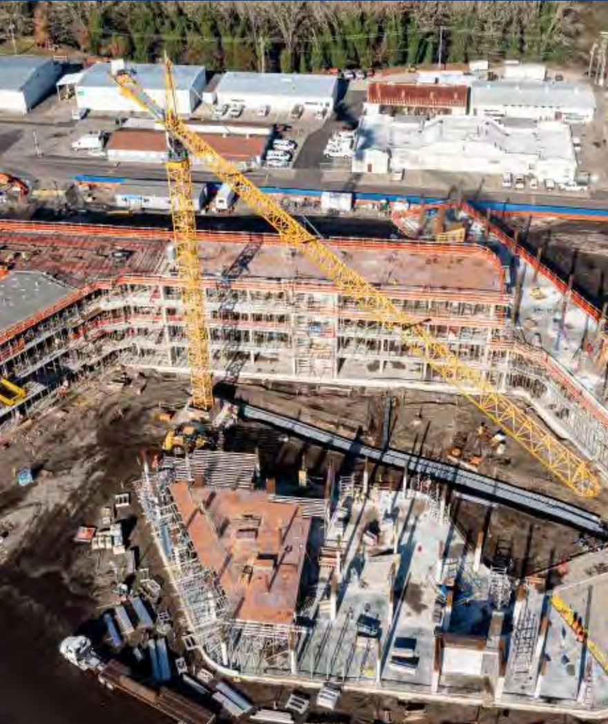
Western State Hospital forensic hospital construction
