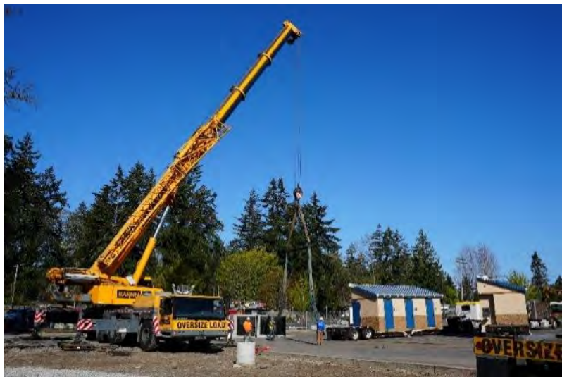
Restroom Construction at American Lake Park
