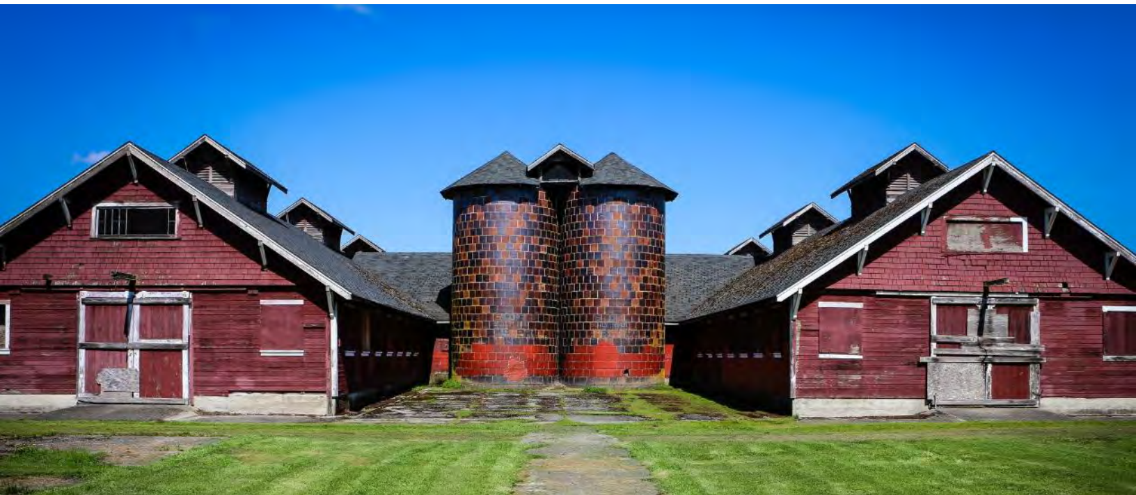
Historic barns and silos at Fort Steilacoom Park
